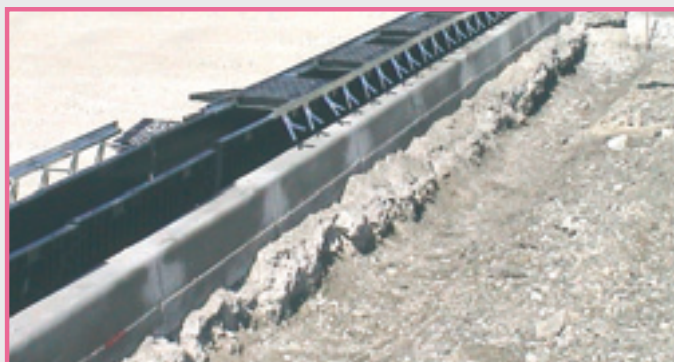
(FIG. 1) • MUFLEDRAIN INSTALLATION UNDERLYING LAYER
